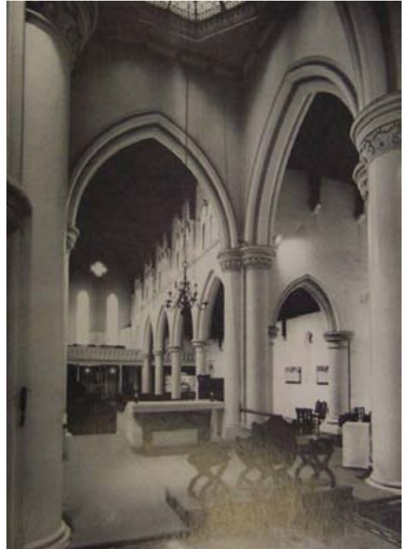
Fig. 28 Interior of the church, 1973 (Survey of London).
