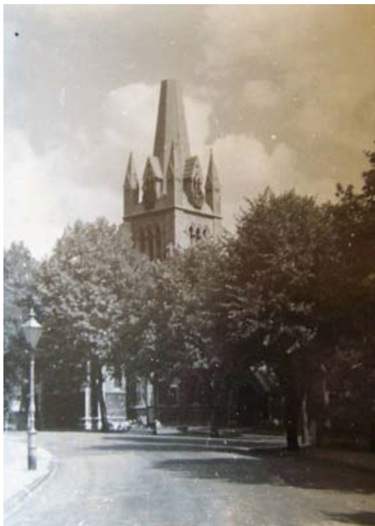
Figs. 18-19 St John's Church in 1942, shorn of a portion of its spire following bomb damage (CCC). The top 26ft of the spire was rebuilt in 1957 (Survey of London).
